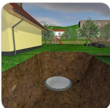
The plastic waste water treatment plant must be situated on the blinding concrete (baseplate) of a thickness of either 100 mm or 150 mm depending on specific type of WWTP reinforced with reinforcing net. A concrete slab is cast on the pre-compacted gravel bed. The required flatness of the blinding concrete is 2 mm/2 m.
