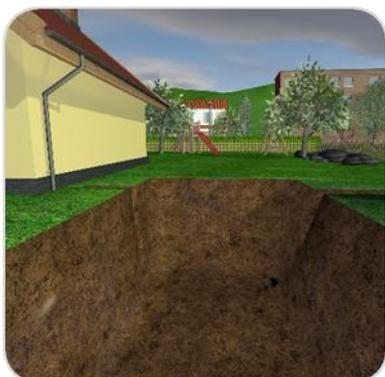
Building pit must be excavated in advance for WWTP installation according to the constructional readiness for specific WWTP type. Execution and security of the excavation must meet the safety requirements. Next, a minor trench should be excavated to allow building of the sheltered area, for example, a wooden house to accommodate the WWTP operation control system (see the figure on the left).
